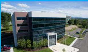
105 West View Rd. 77,000 sq.ft. of office space
